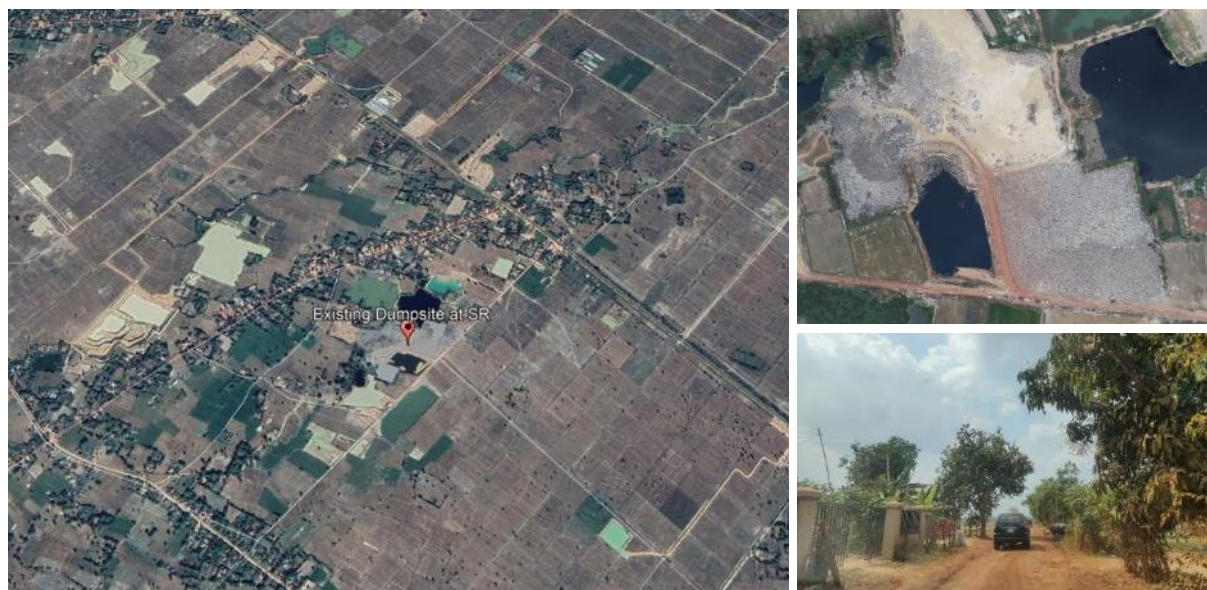
Figure 3.3-1: Existing Dumpsite in Anlong Pir Village, Trapeang Thom Commune
